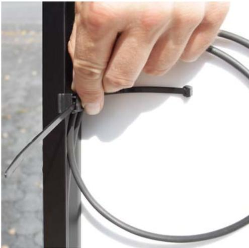
Lay the cable all the way to the solar module. Use one of the edge clips supplied to attach it to the module frame below the target measuring point to prevent rain water from penetrating into the STS.
